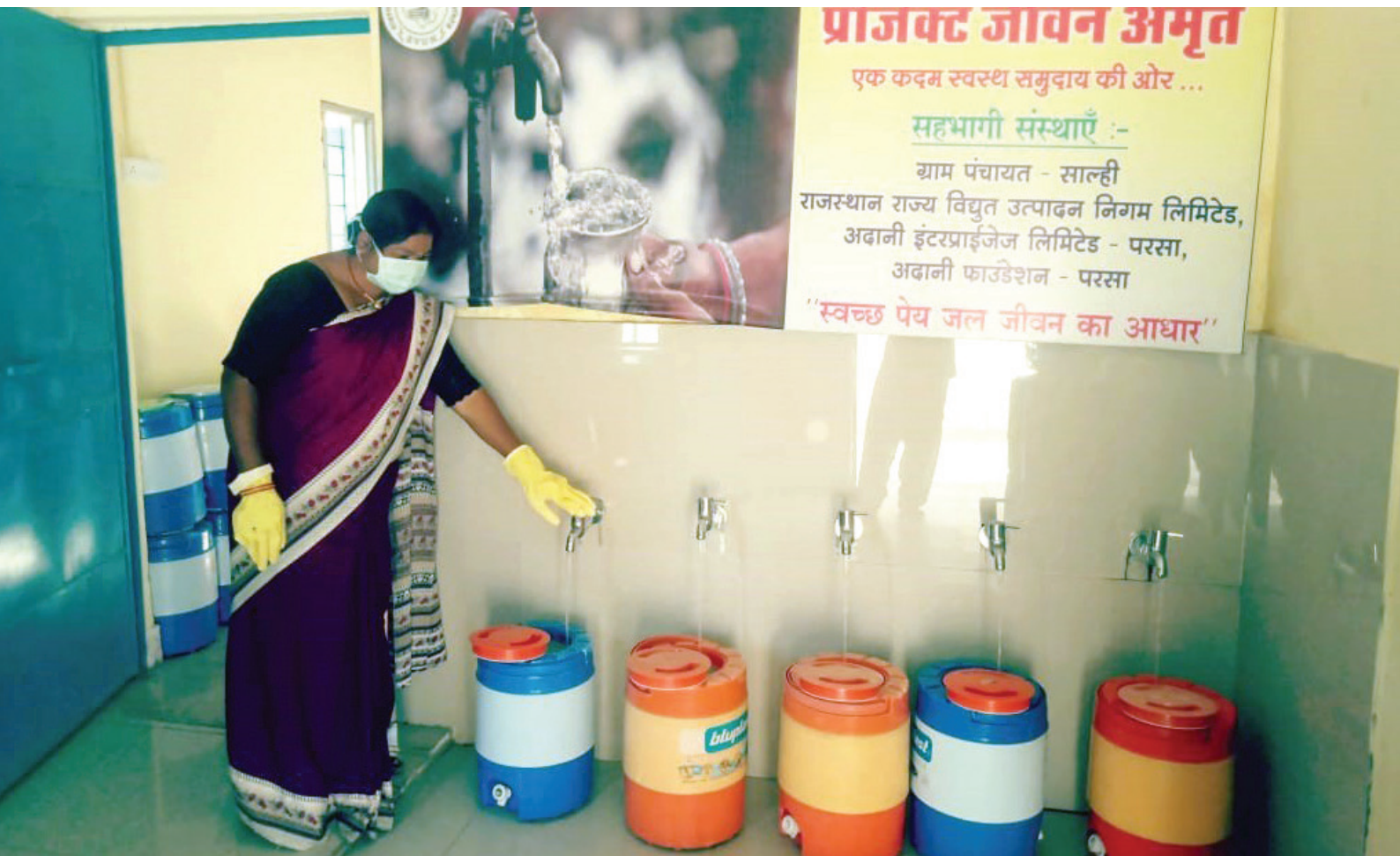
Project Jeevan Amrit – Water treatment unit
