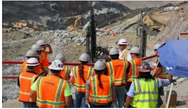
Construction at site
