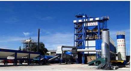
Contractor Camp Mobilization
