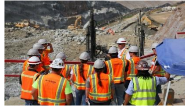
Construction at site
