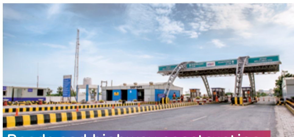
Roads and highway construction
